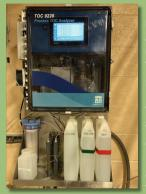
In 2023, Metro Water Services installed new on-line Total Organic Carbon (TOC) analyzers (YSI 9220) at both the Omohundro and K.R. Harrington Water Treatment Plants for continuous monitoring of raw and finished water.
